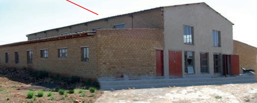
Children's Dorm & Dining Facility
